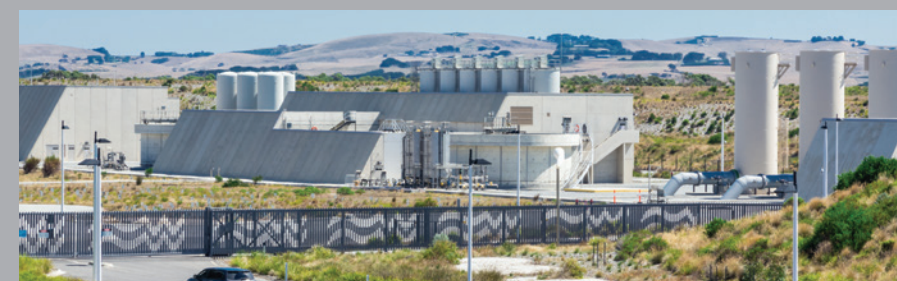
The Victorian Desalination Plant, in the state of Victoria, Australia was completed in 2012 with an estimated output of 410 megalitres of water per day.
